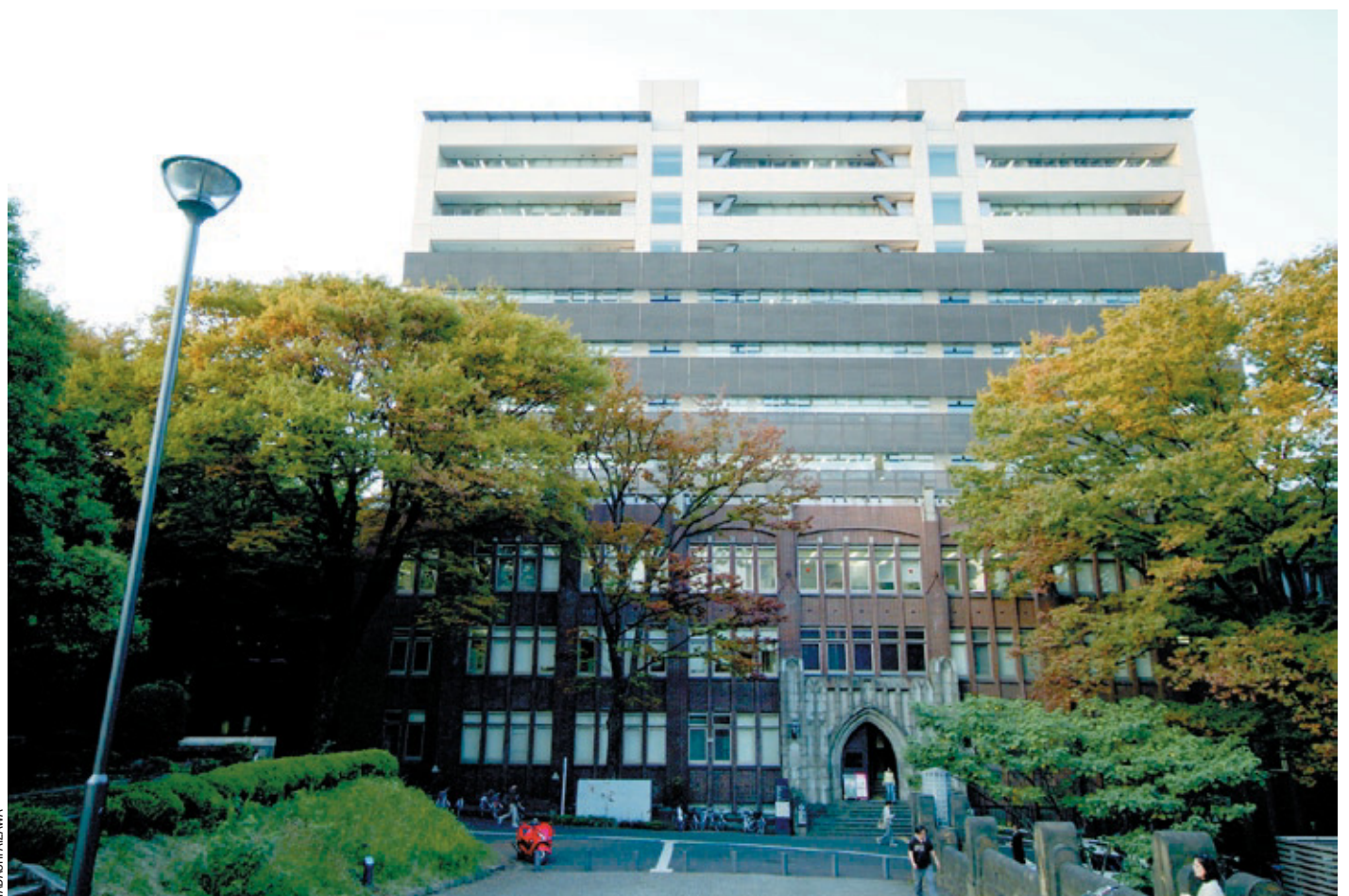
The test bed: Building No. 2 of the Faculty of Engineering
